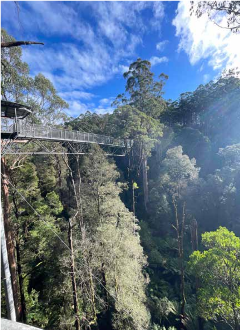
The cantilevered walkway above Young Creek at the Otways Fly
